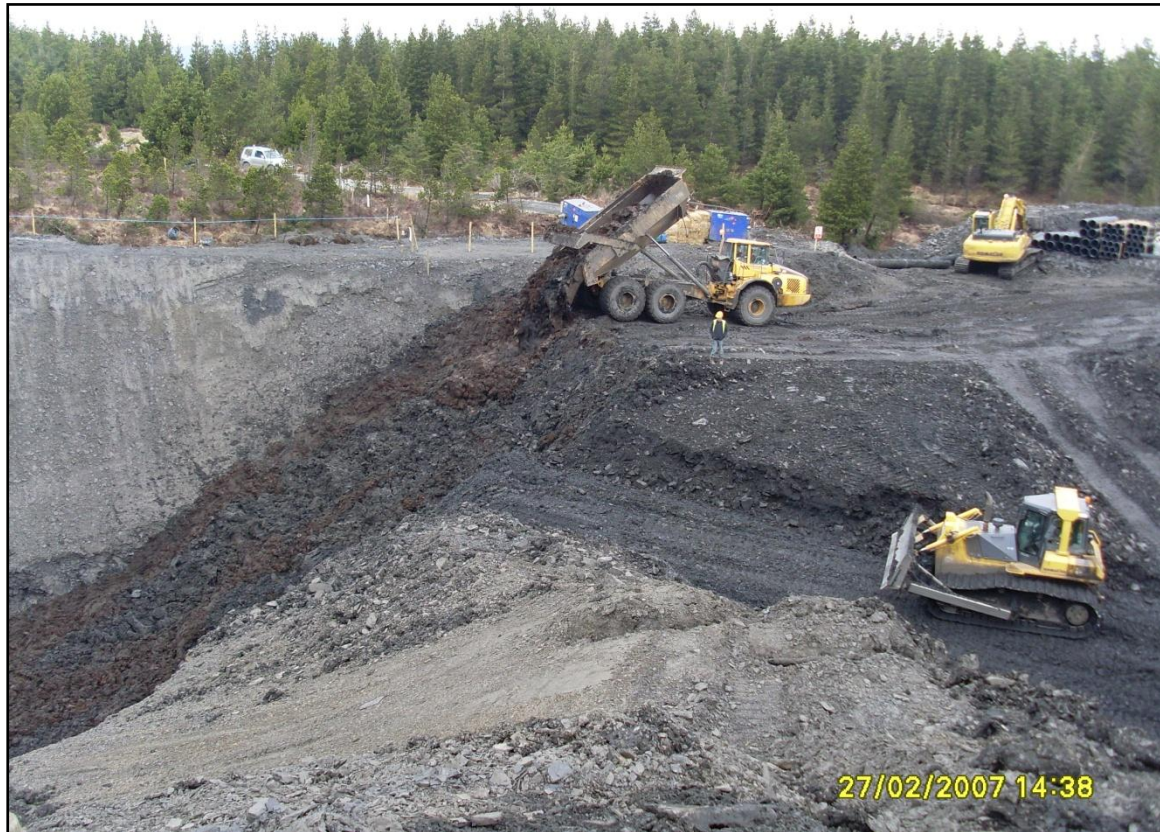
Photo No. 2.3.2 - Backfilled peat repository
