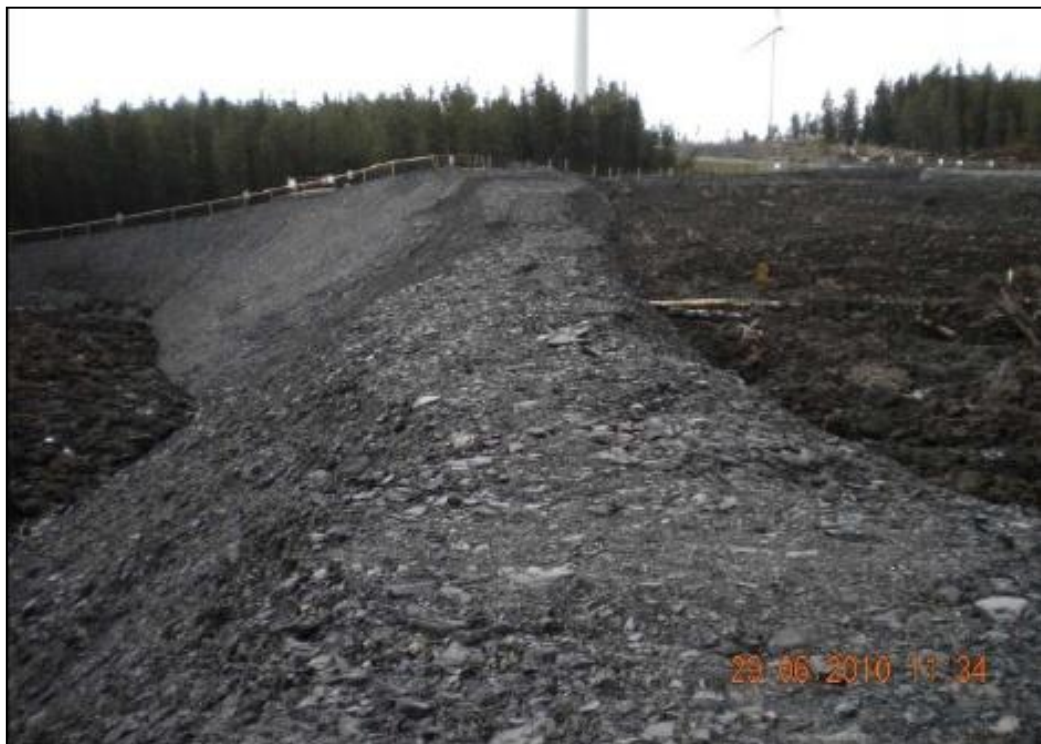
Photo No. 2.3.3 - Deep banded peat repository approximately 2.5 years after filling
