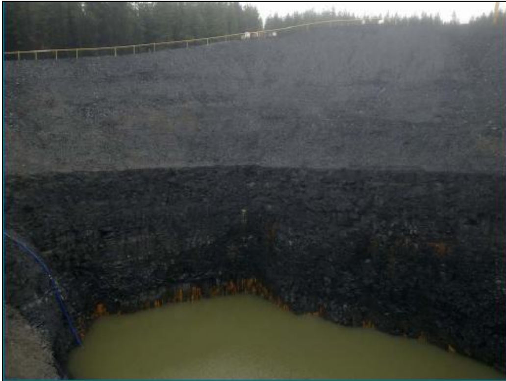
Photo No. 2.3.12 - Completed deep borrow pit in rock
