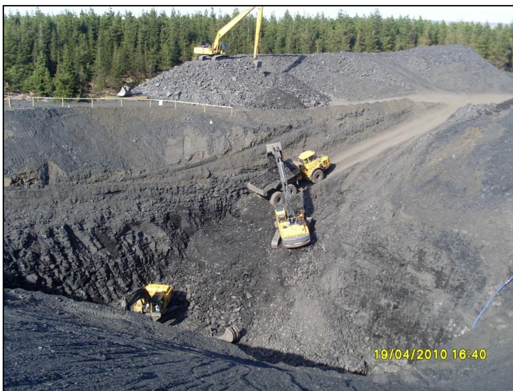
Photo No. 2.3.11 - Excavating a deep borrow pit in rock
